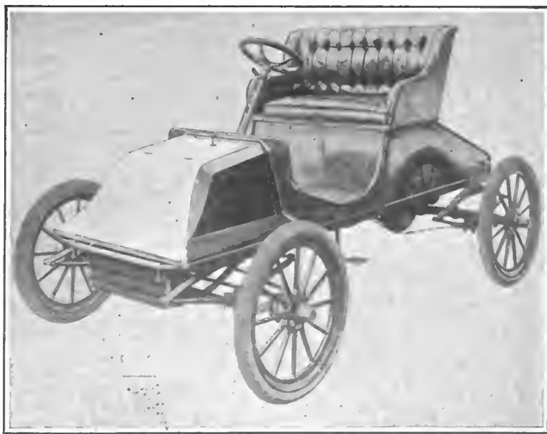
GALE LIGHT CAR FITTED WITH SINGLE CYLINDER HORIZONTAL MOTOR.
